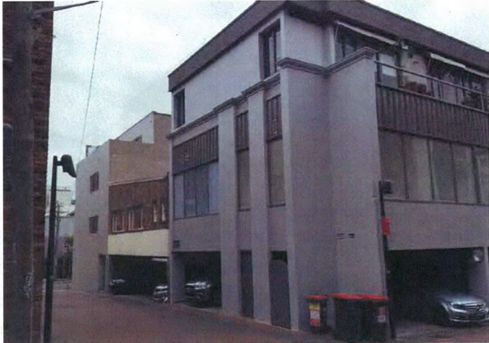
View west down Pole Lane from Hume Lane
