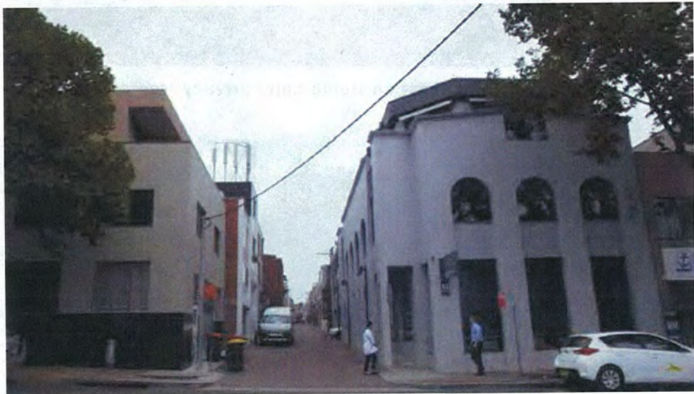
View south on Hume Lane with rear of Willoughby Road properties
