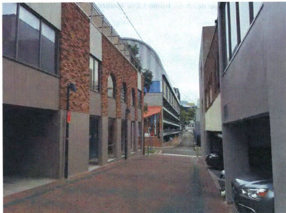
View west down Pole Lane towards Hume Street carpark
