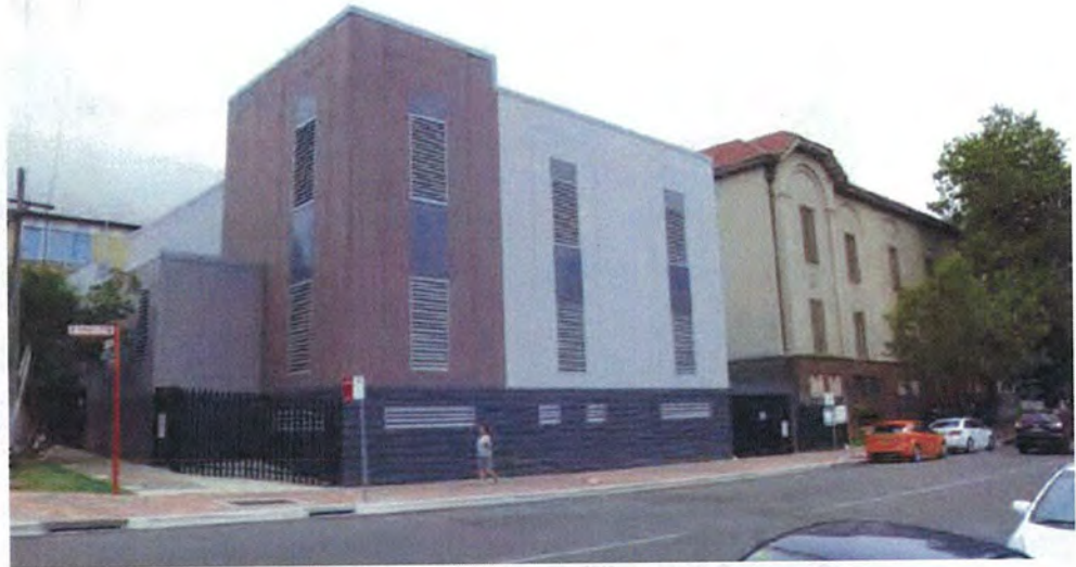
View west on Albany Street of substation complex
