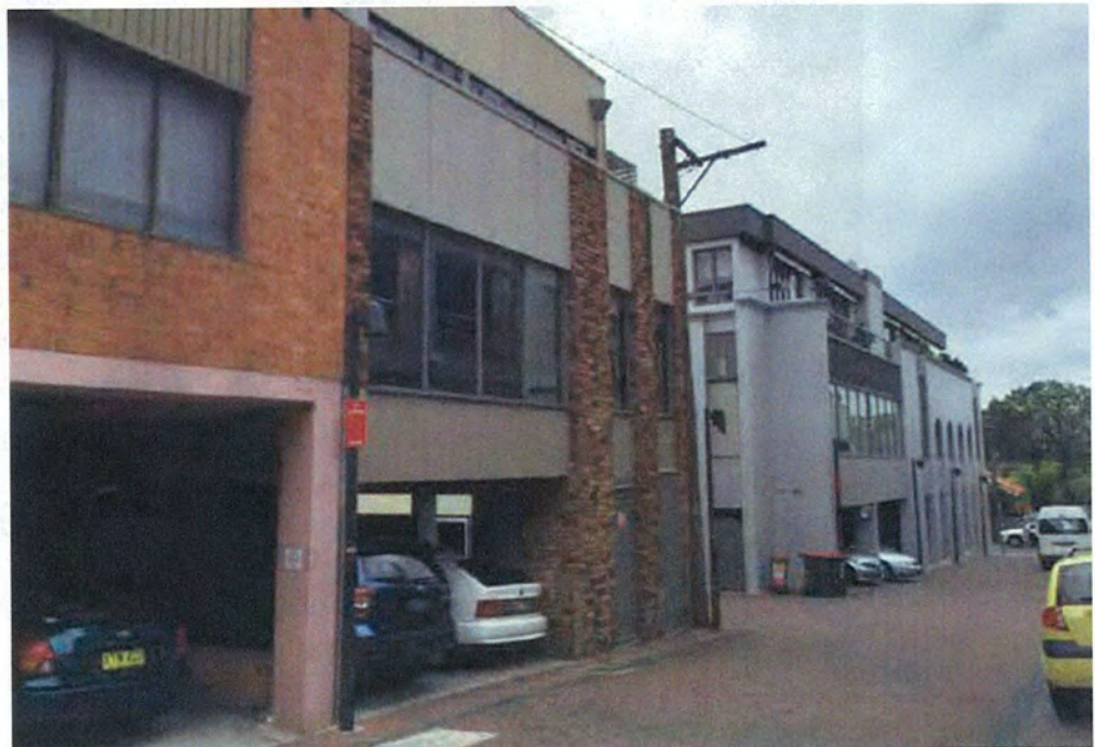
Hume Lane frontage view north-west
