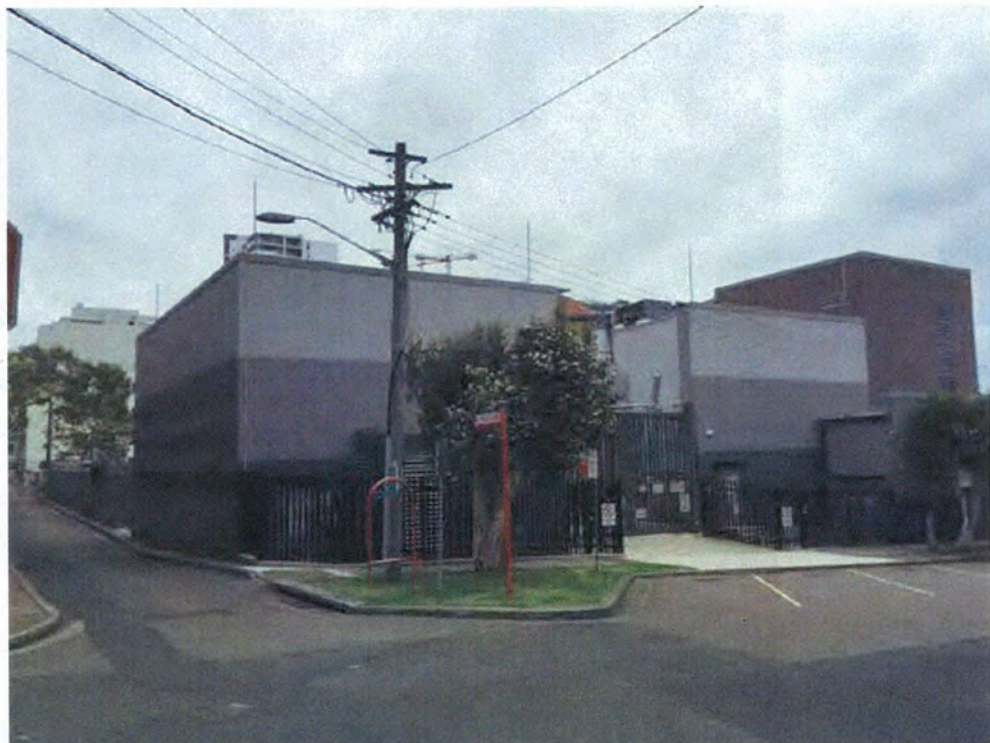
View west on Hume street of substation complex
