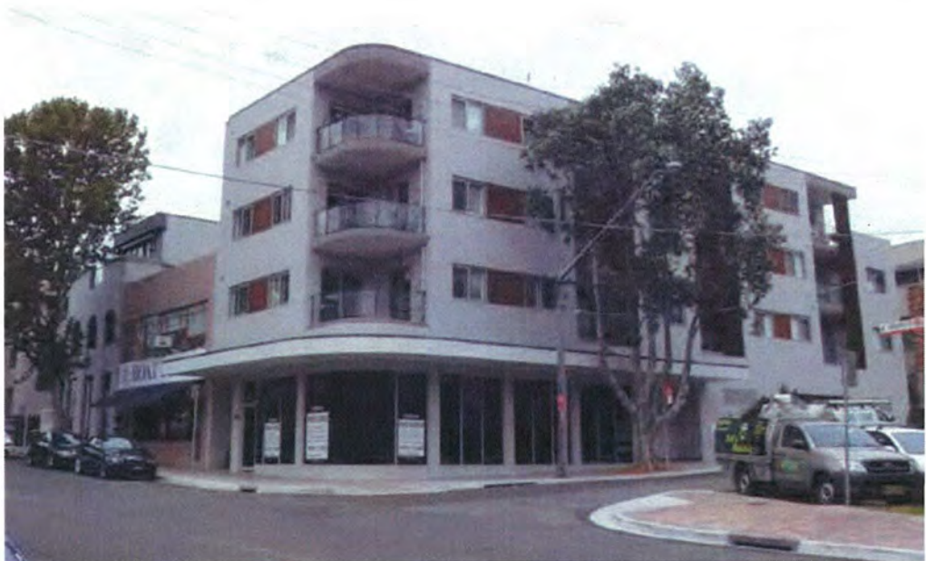
29 Albany Street mixed use development to the west
