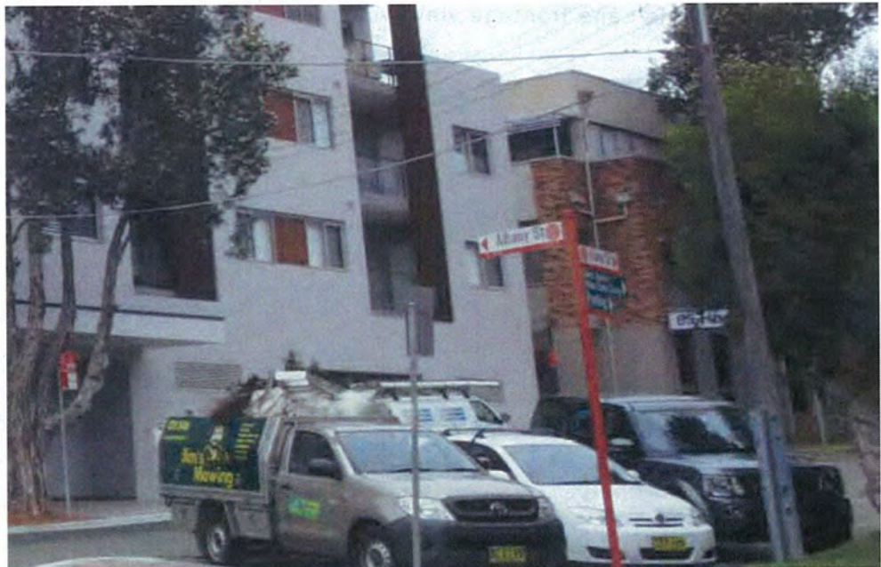
Hume Street frontage view south-east
