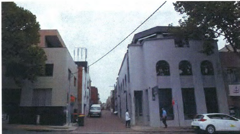
View west down Hume Lane
