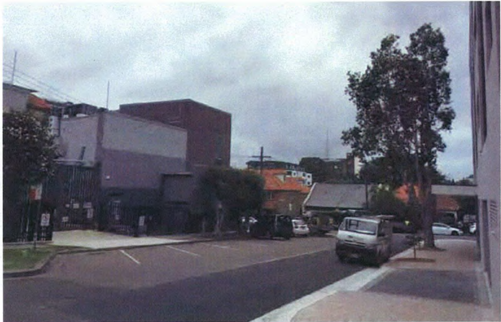
View north-west on Hume Street towards Albany Street and substation complex
