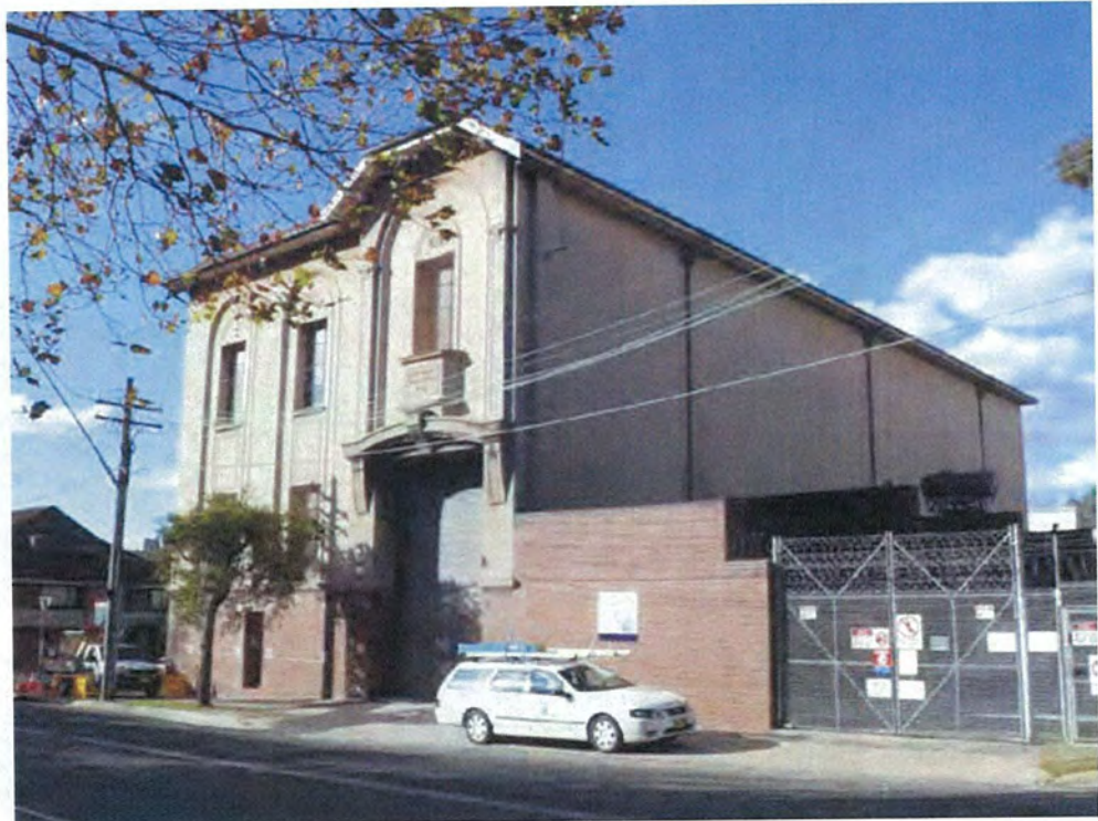
View of 23 Albany Street from the south-west
